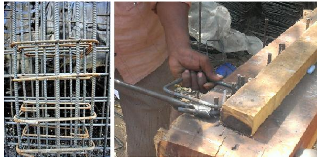
Figure 2. Manual Stirrup bending operation
