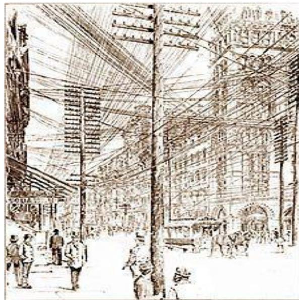
Fig.2 Multiple transmission lines were required for different voltages.
